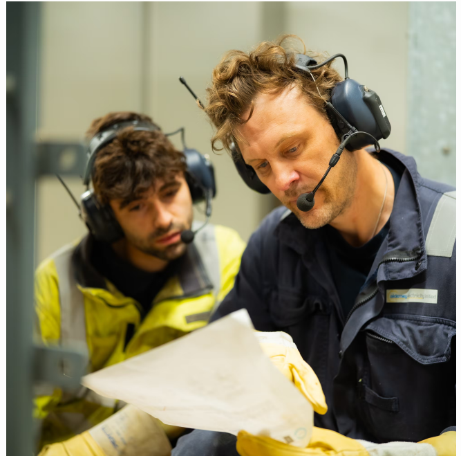
Alderney Electricity technicians at work.
